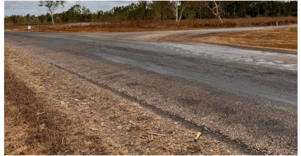
Figure 4-3.3: Keith Venables Road Sealed (top) and Unsealed (bottom)
